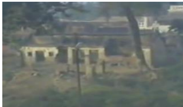
Fig 1.10 The demolished structure
