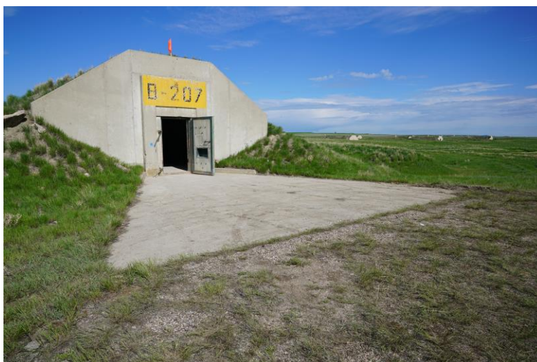
Fig. 1: Bunker B-207, one of 507 concrete bunkers at Vivos xPoint being retrofitted for future disaster.
